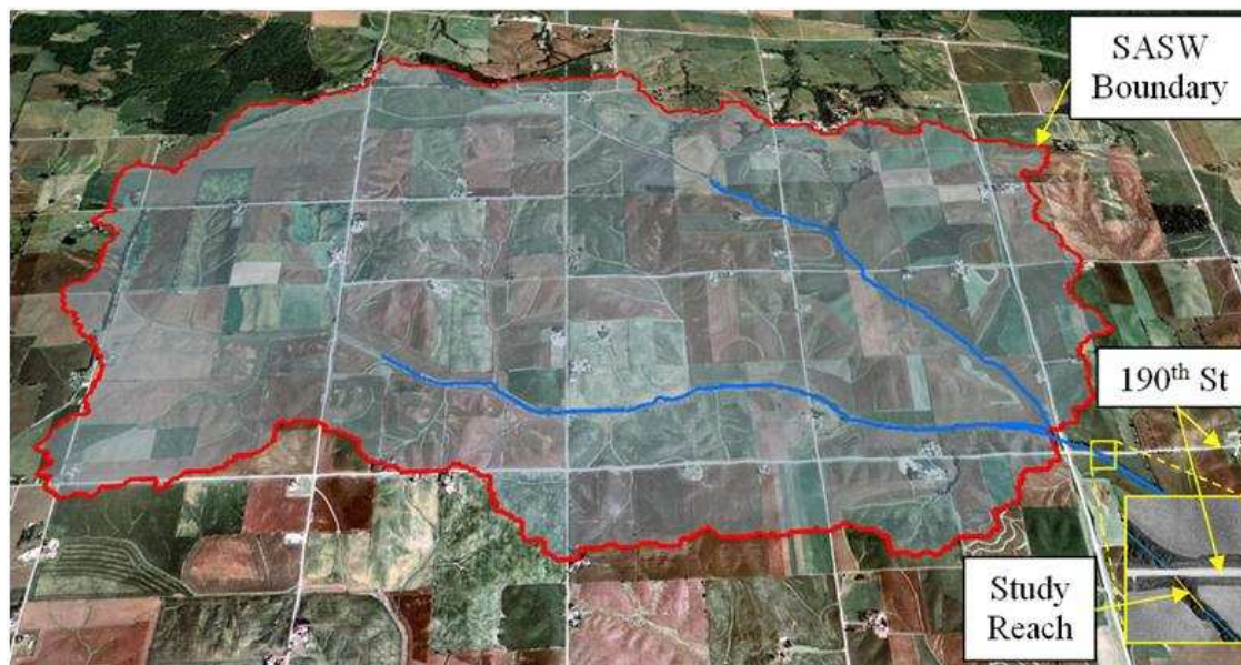
Figure 3.2. Aerial view of the SASW
